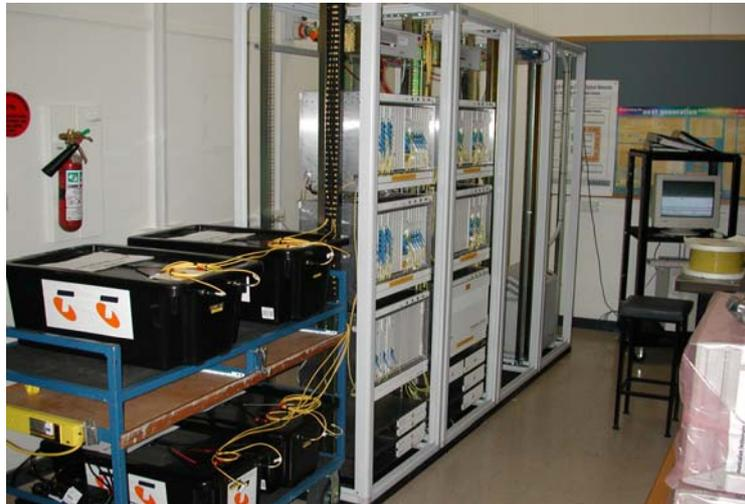
*Figure 73 The Siemens TranXpress Multiwavelength Transport System*
